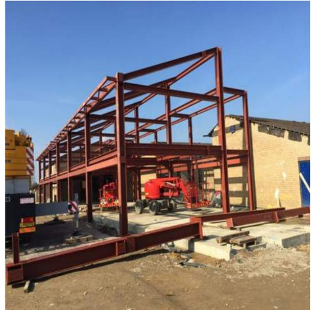
As you can see from the pictures, the building work is progressing at some pace. A large part of the groundwork has been completed, and the steel frame has started to go up. The steel frame is delivered on large flatbed trucks, outside of school hours, and an extremely large crane lifts each section into place, before being secured by builders either on the ground or high in the air as the picture below demonstrates!
